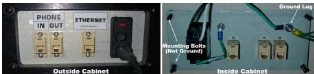
Figure 46. AC Power Plate (Standard Cabinet)
